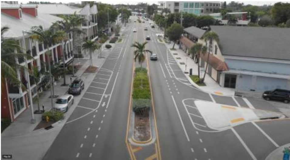
Figure 8. Wilton Drive, Broward, FL after conversion from 5-lanes to 3-lanes (Credit: Road Safety Foundation)
