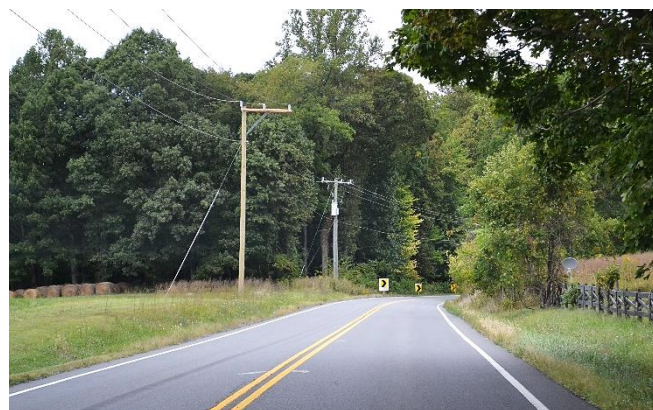
Regular Width Edge Line Pavement Markings (Example Location: Route 9, Loudoun County, VA)
