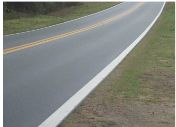
Wider Edge Line Pavement Markings (Example Location Source: Texas Transportation Institute)
