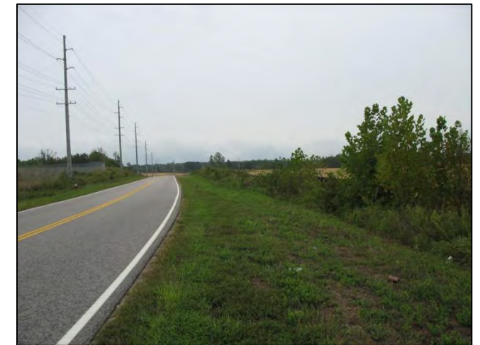
Graded shoulder available in CC Industrial Park.
