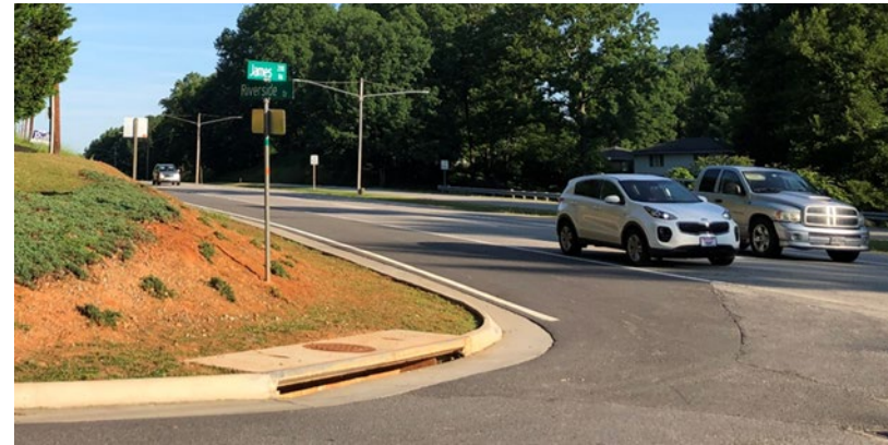
FIGURE 38: JAMES ROAD INTERSECTION. THE EMBANKMENT AT THE SOUTHWEST QUADRANT SHORTENS SIGHT DISTANCE FOR DRIVERS LOOKING WEST FROM THE NORTHBOUND APPROACH.
