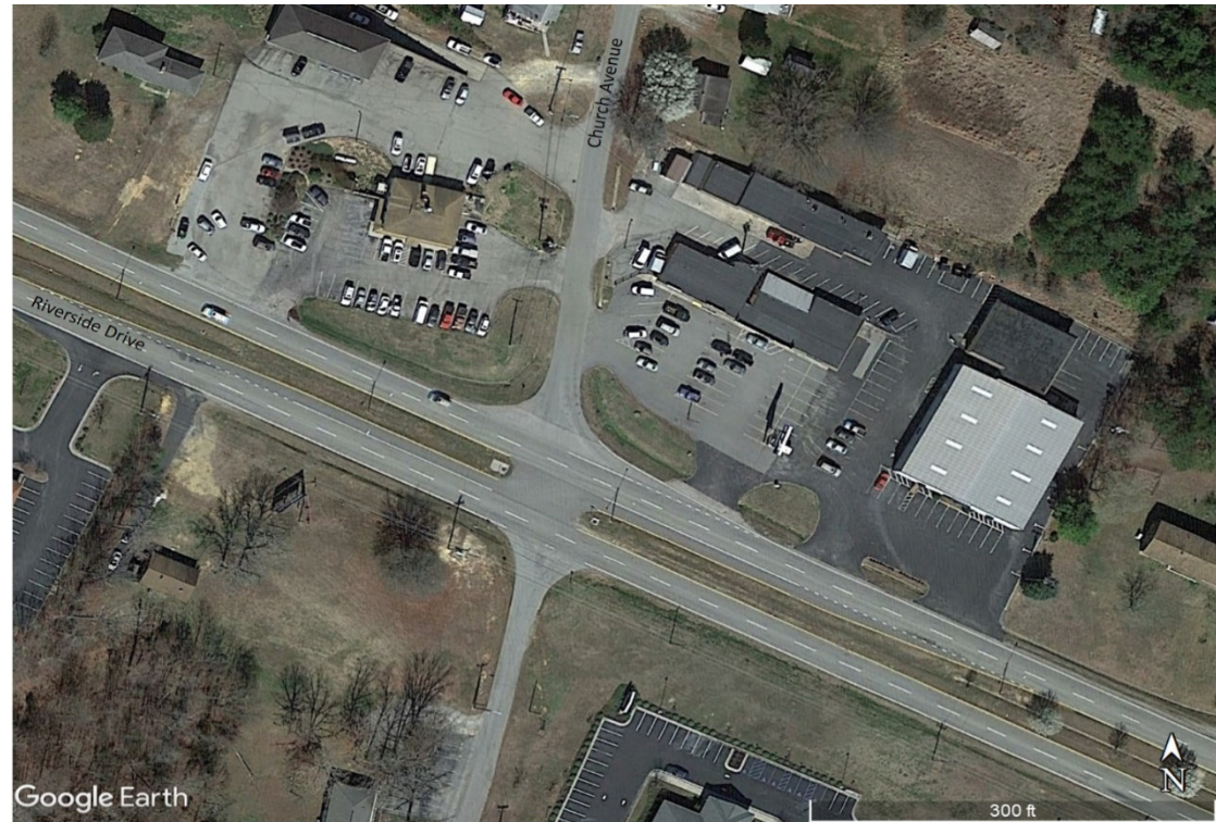
FIGURE 33: ENTRANCE SPACING AT CHURCH AVENUE. SUCCESSIVE ENTRANCES DO NOT MEET VDOT SPACING STANDARDS.
