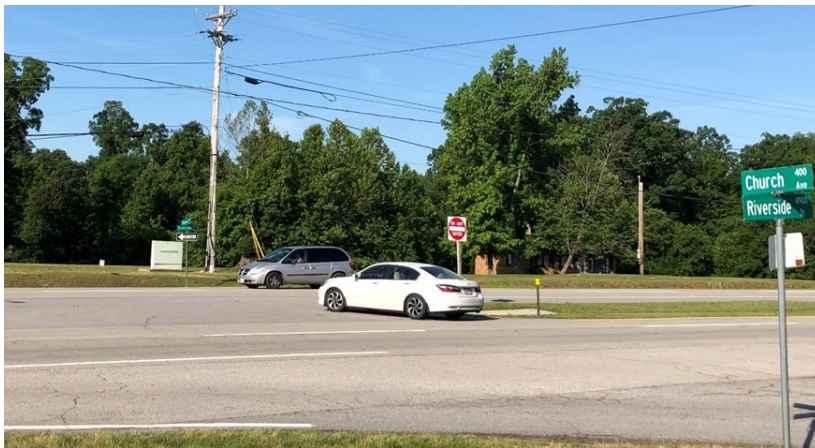
FIGURE 41: VEHICLE WAITING IN MEDIAN AT CHURCH AVENUE. THE MEDIAN STORAGE WIDTH AT SEVERAL INTERSECTIONS IN THE EASTERN PORTION OF THE STUDY AREA IS NARROW, MEASURING 20 FEET WIDE WITH AN 11-FOOT LEFT TURN STORAGE LANE, FOR 31 FEET OF VEHICLE STORAGE.
