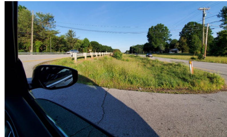
FIGURE 37: ELEVATION DIFFERENCE AT STONY MILL ROAD. EASTBOUND US 58 IS HIGHER THAN WESTBOUND, MAKING IT DIFFICULT FOR WESTBOUND LEFT TURNING VEHICLES TO ACCELERATE FROM A STOP.
