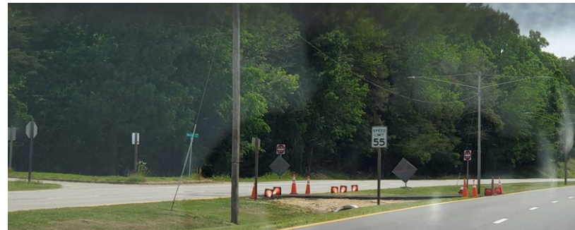
FIGURE 39: MEDIAN OPENING AT BEECH AVENUE. THE NEWLY PAVED MEDIAN OPENING ALLOWS LEFT TURNS FROM BEECH AVENUE ONTO EASTBOUND US 58, BUT EASTBOUND VEHICLES ON US 58 CANNOT MAKE A LEFT TURN INTO BEECH AVENUE.
