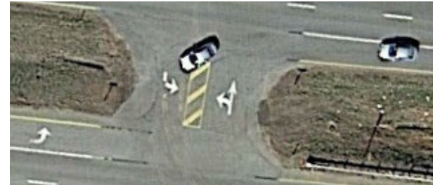
FIGURE 60: MEDIAN PAVEMENT MARKINGS AT BROSVILLE INDUSTRIAL PARK ROAD. A SIMILAR PAVEMENT MARKING SCHEME IS RECOMMENDED AT THE INTERSECTION OF OAKWOOD DRIVE.
