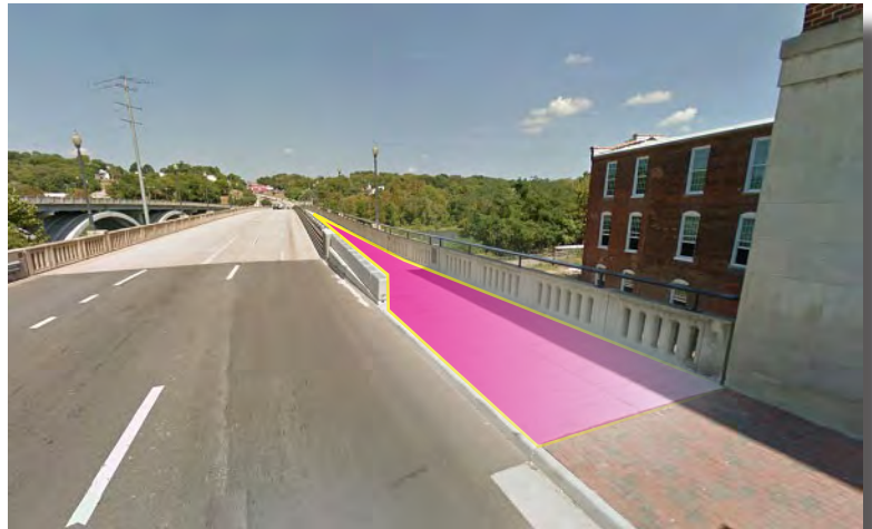
The separated bridge pathway, highlighted in pink in the image above, provides a safe route across the Dan River for bicyclists and pedestrians alike.
