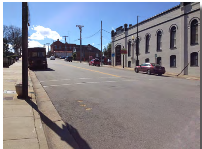
Crosswalks marked with thin white lines, such as this example on Patton St shown above, have low visibility for drivers.
