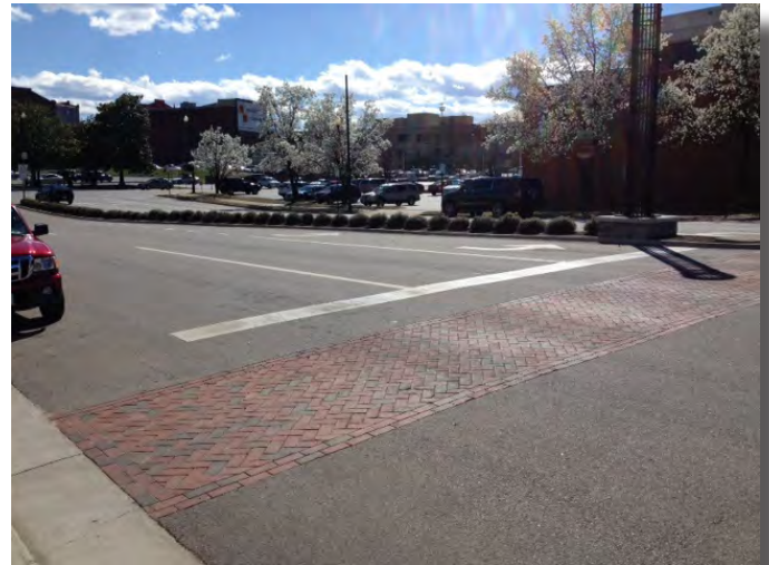
Brick crosswalks can be difficult for drivers to distinguish from the surrounding pavement.
