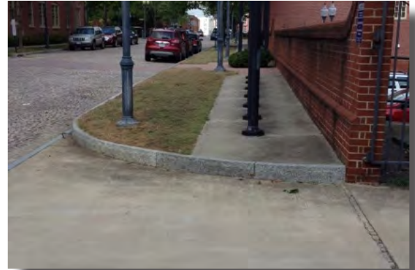
This sidewalk on Bridge Street lacks curb ramps and also is obstructed by flag poles.
